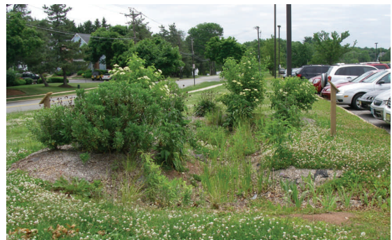
Typical rain garden adjacent to parking lot
