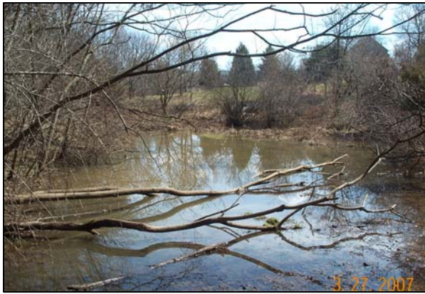
Poorly Maintained Detention basin at Country Acres
