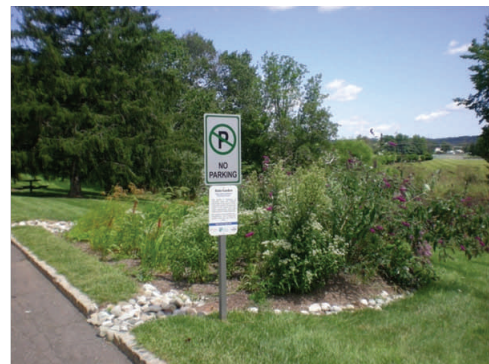
Typical rain garden adjacent to parking lot
